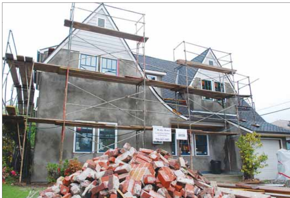
The exterior of the Mortensen residence during construction
