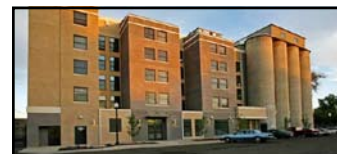
Figure 10 - Completed New Building 2, 2008 photo by Cathy Kelley
