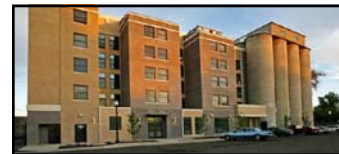
Figure 10 - Completed New Building 2, 2008 photo by Cathy Kelley
