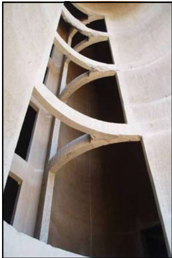
Figure 6 - Openings in Silo
