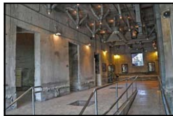
Figure 7 - New Ground Floor Lobby in South Silos courtesy of Michael Malinowski, AIA
