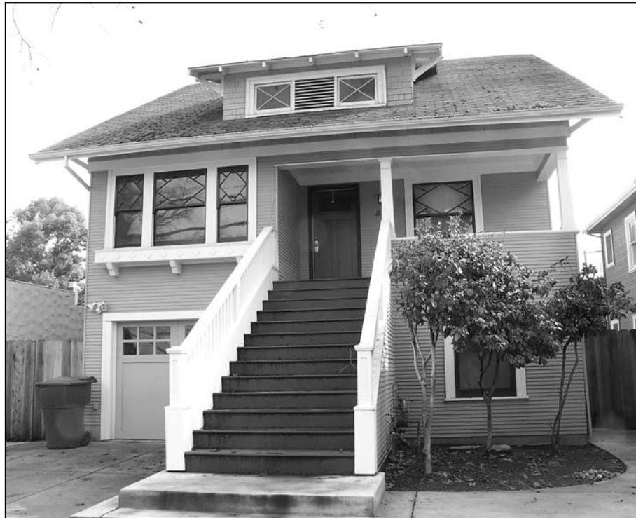
This home was raised and moved back on the lot and a basement apartment was added
