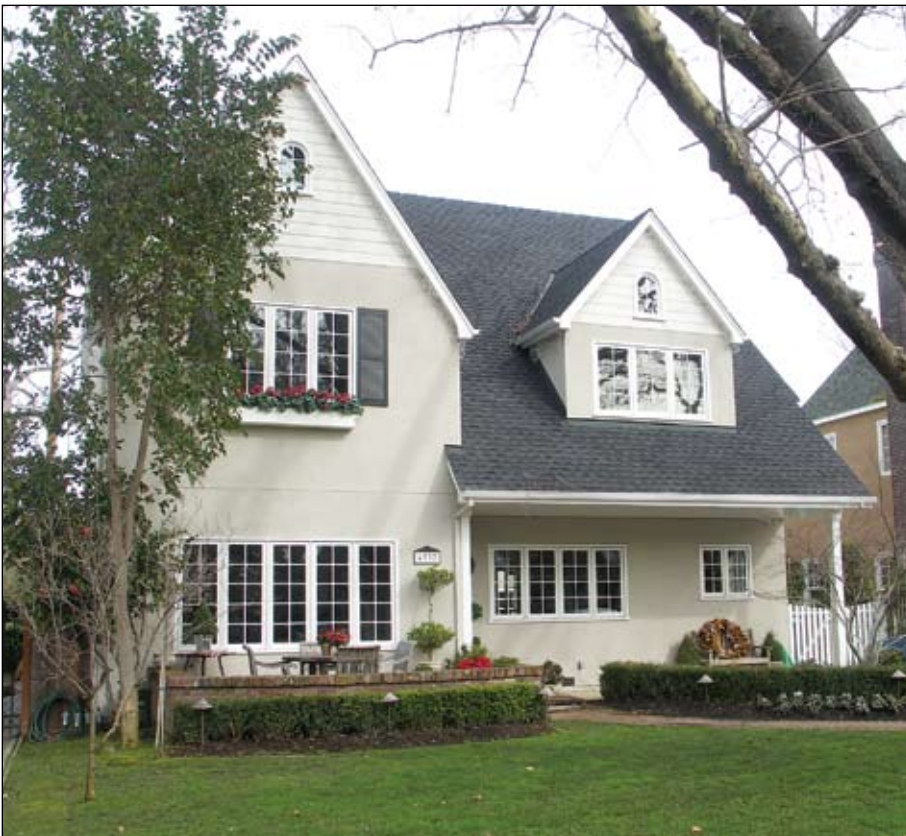
A second story was added to this East Sacramento home
