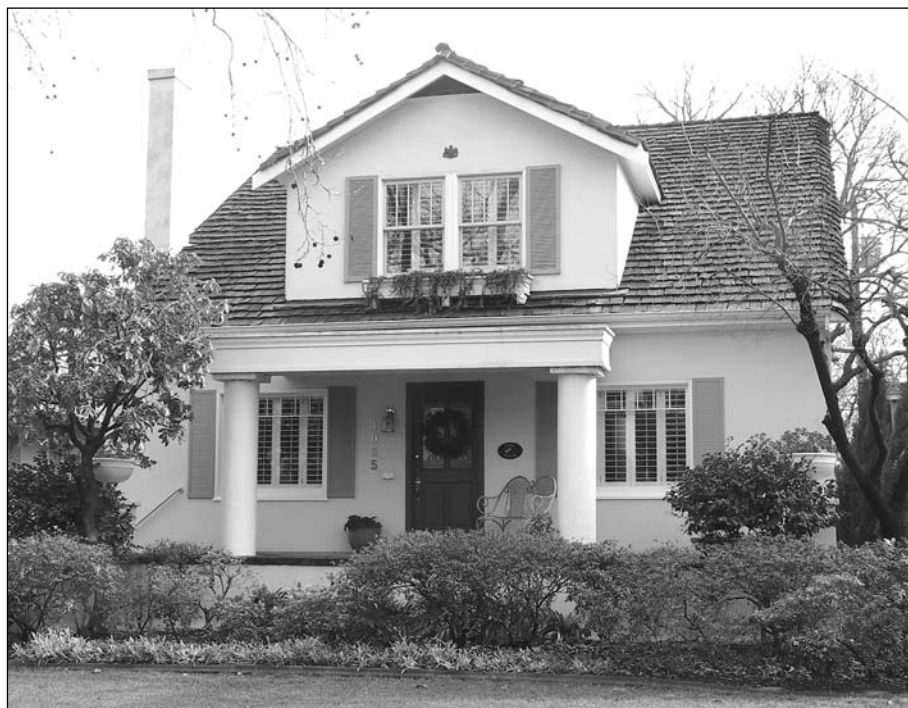
A second story was added to the back of this house
